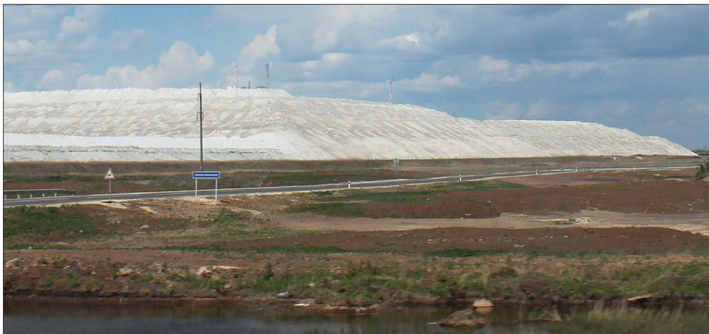
Phosphogypsum is commonly stock in large open areas a by-product from the phosphate fertilizer industry.
